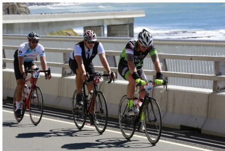
Cycling on the Sea Cliff Bridge, Source: KPMG, 2016
