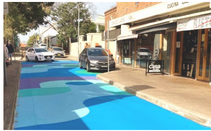
Painted road treatments at Bligh Street, Kirribilli, North Sydney, Source: KPMG, 2021
