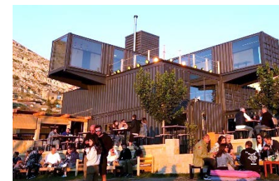
Pop-up hotel and bar in Faraiya, Lebanon utilising shipping containers, Source: KPMG, 2019
